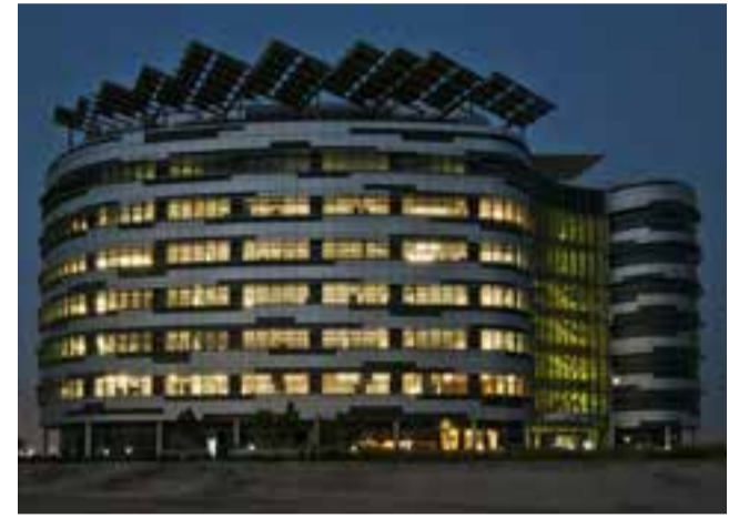
IRENA Headquarters in Abu Dhabi (Photo: woodsbagot.com)
